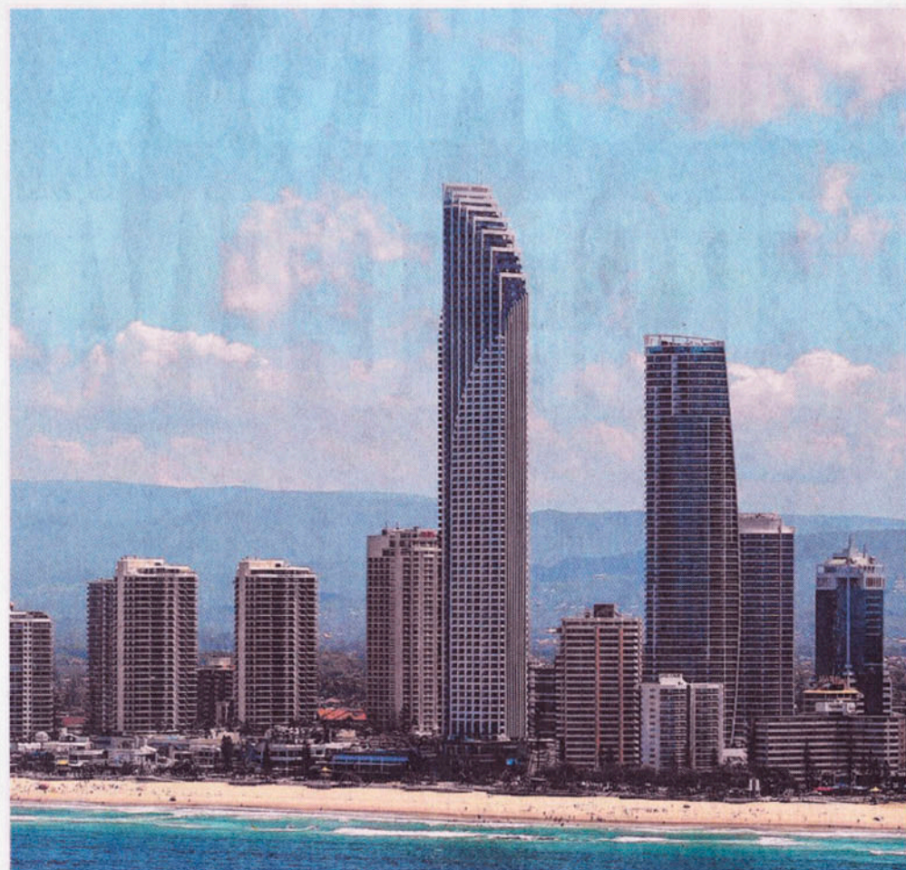
The 77-level Soul Surfers Paradise tower, centre
